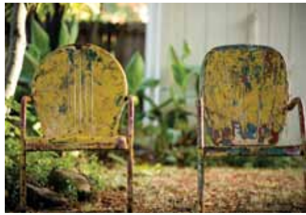
► Condition of Surface Prior to Painting
